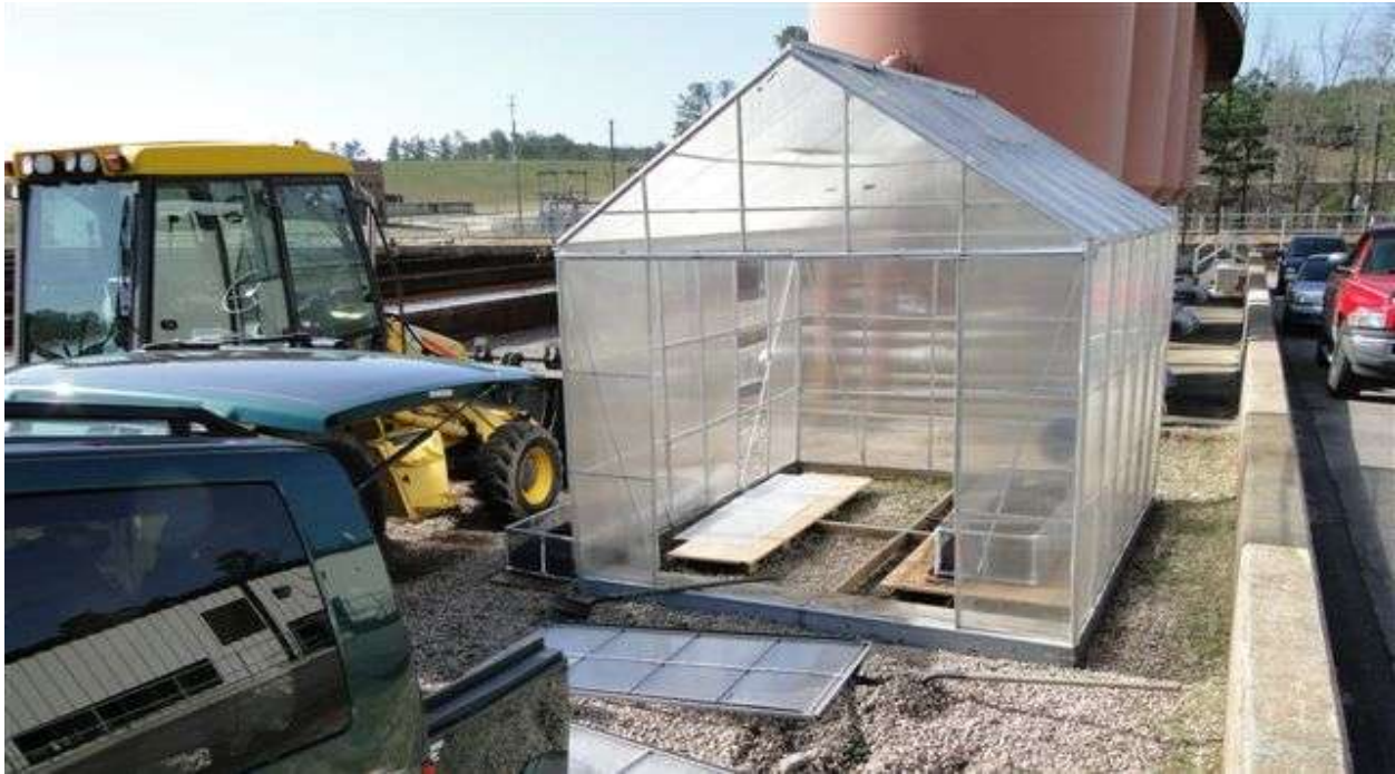
Figure 2.7 Field pilot test set up at E.M. Johnson WTP in Raleigh, North Carolina
