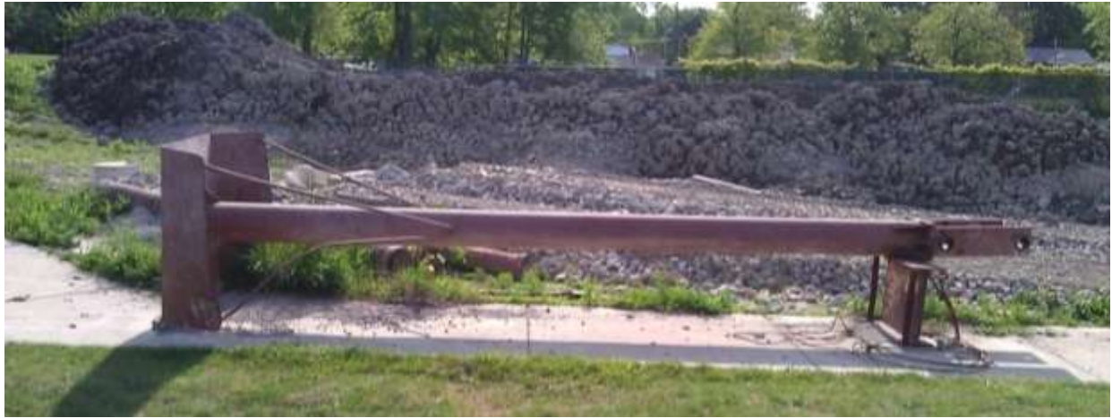
Figure 4.12 Extension arm fabricated by Mentor On-the-Lake WTP mechanics to till over sludge lagoon residuals
