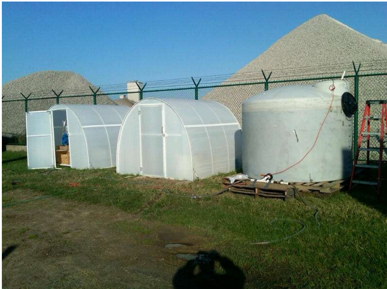
Figure 2.6 Field pilot test set up at Morgan WTP in Cleveland, Ohio
